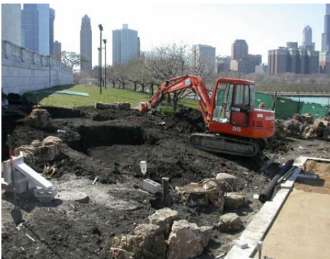
Excavating the waterfall area.
