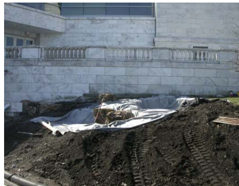
Laying liner for the 80-foot waterfall.
