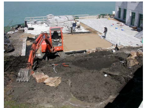
Patio installed while excavation begins.
