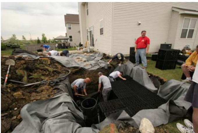
Forty modular AquaBlox® set into excavated storage basin after liner is laid into place. Up to 1300 gallons can be stored underground.
