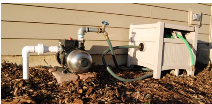
Plumbing from the Downspout Filter runs to the reservoir.
