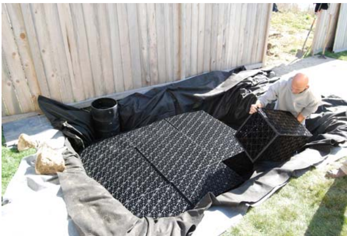
AquaBlox® are placed into the excavated reservoir.
