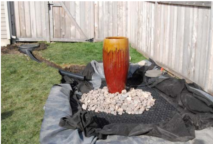
Plumbing from the Downspout Filter runs to the reservoir.
