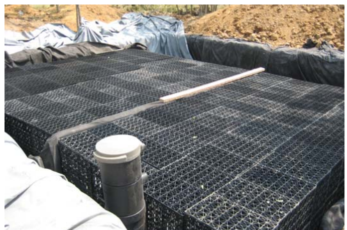
Two chambers are created. The first holds the initial roof run-off and the second holds the sterilized water.
