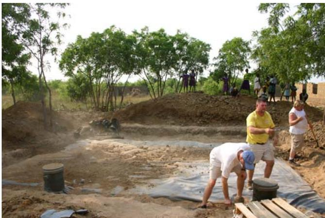
Two feet of soil is mounded over the reservoir to block water born contaminants from entering the basin.
