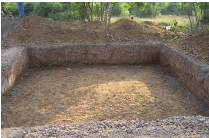
The 22' x 24' basin has a depth of 4 feet. 240 AquaBlox® Water Matrix units will fill this hole.
