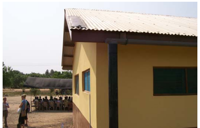
A solar panel was installed on the roof of the school in order to power the transfer pump.
