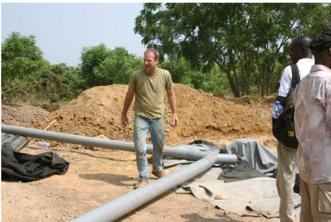
Underground pipe is installed to carry water from the downspout to the rainwater storage basin.
