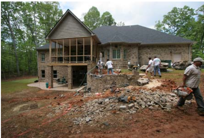
Homeowner property before the RainXchange™ System and Pondless® Waterfall are installed.
