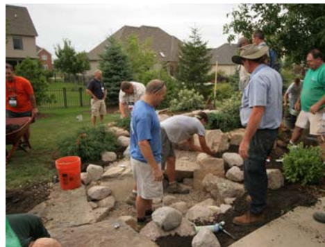
During construction of the waterfall and rainwater harvesting system.
