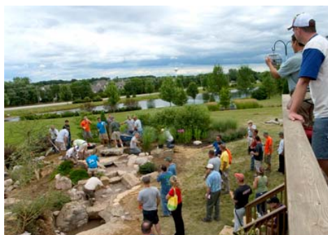
During construction of the waterfall and rainwater harvesting system.
