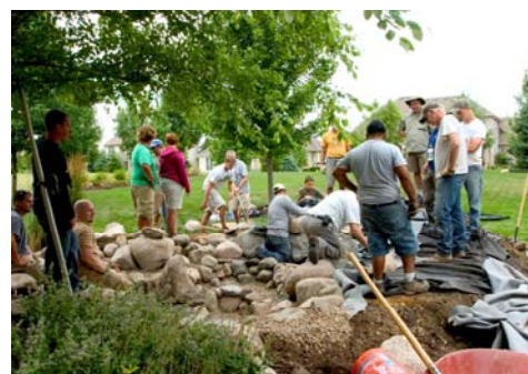
Liner and rock are placed to form the stream and waterfall.
