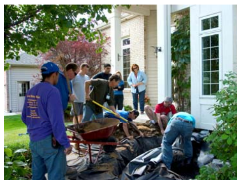
Liner is spread before the AquaBlox® D-Raintanks® are placed.
