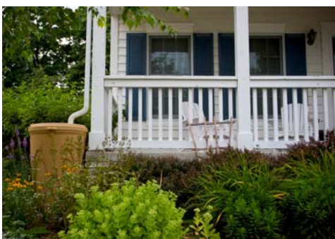
RainXchange™ Rain Barrels installed throughout the neighborhood.
