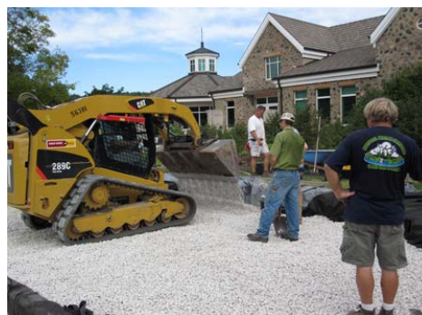
Aggregate layer added before pavers
