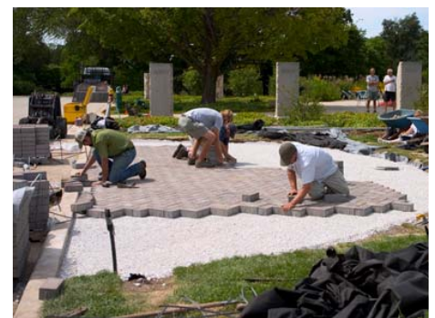
Laying the permeable pavers
