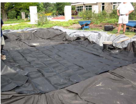
Woven geotextile set over AquaBlox® D-Raintanks®
