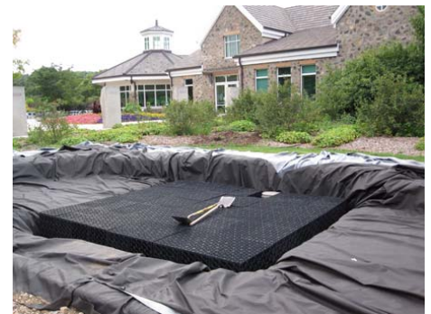
AquaBlox® D-Raintanks® installed.
