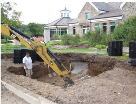
Excavating the reservoir for the patio.
