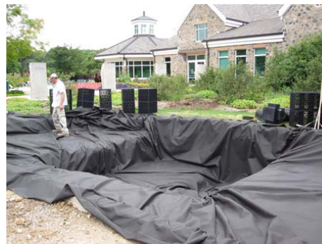
Laying liner for the 500 square foot basin.
