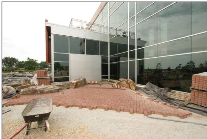
Permeable pavers are laid in place.
