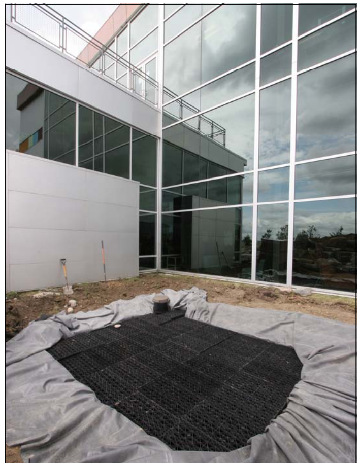
Excavation of site. RainXchange™ modular storage basin will be placed underneath permeable patio.
