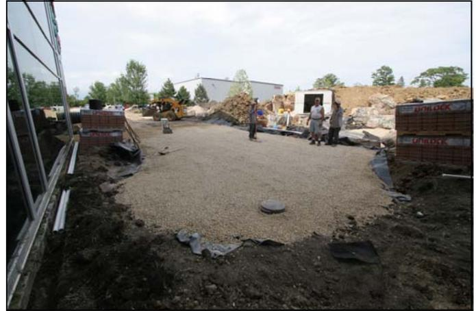
The gravel and screening base is leveled and compacted.
