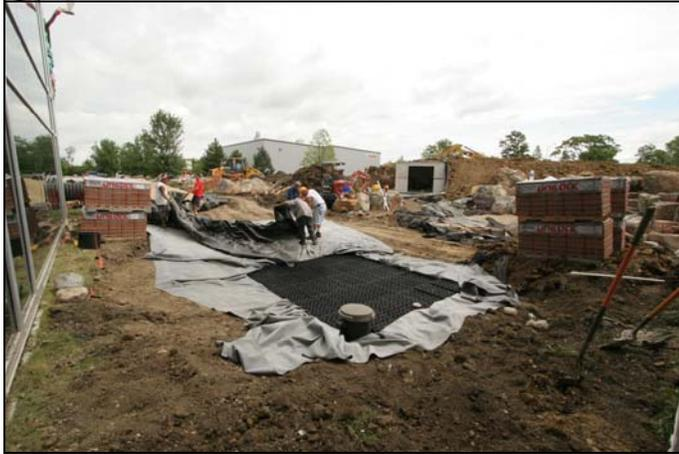
A water permeable woven geotextile fabric covers the top of the AquaBlox® Water Matrix tanks providing a permeable base for the gravel and screening to be spread over the storage system.
