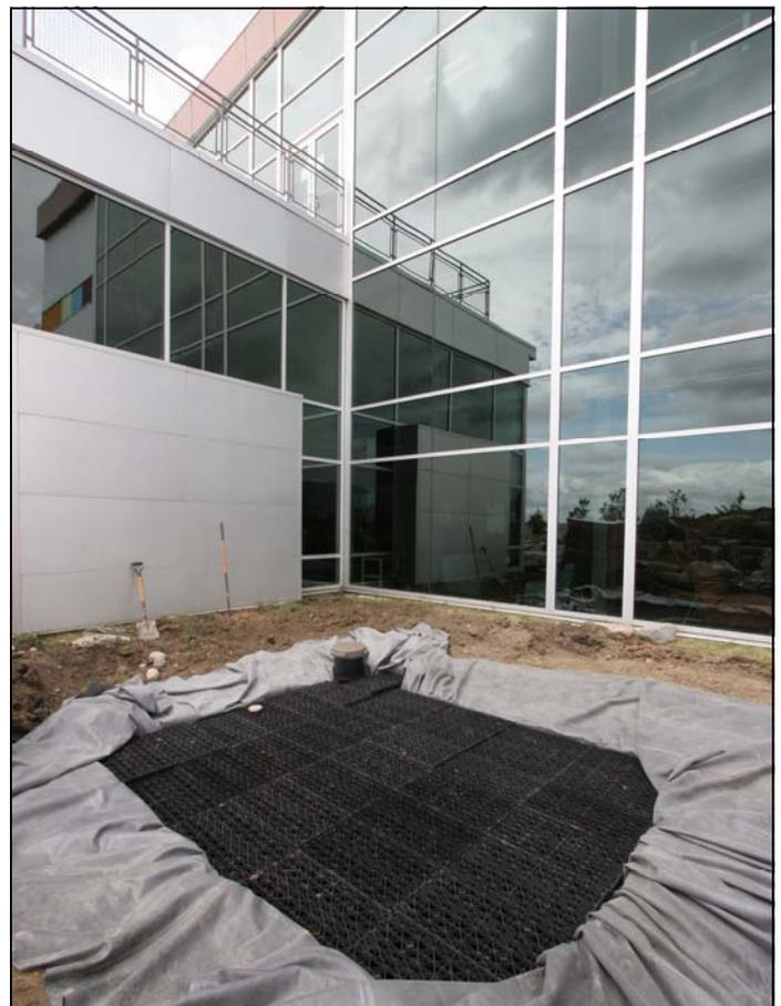
The entire base of the patio is lined with an impermeable membrane to capture the water and direct it towards the water storage basin. 96 AquaBlox® Water Matrix tanks are positioned inside a 9 ft. x 11 ft. x 6 ft. deep basin creating 3,000 gallons of water storage capacity.
