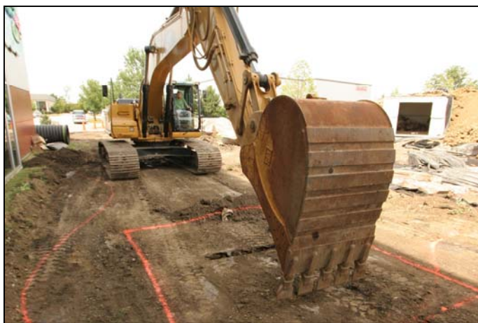
Excavation of site. RainXchange™ modular storage basin will be placed underneath permeable patio.
