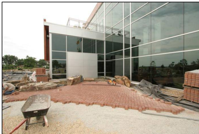
Permeable pavers are laid in place.
