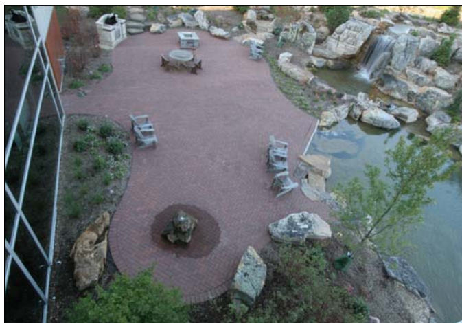
Overhead view of the completed project. Note the fountain rock positioned directly above the AquaBlox® area.
