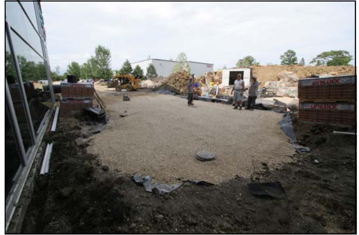
The gravel and screening base is leveled and compacted.
