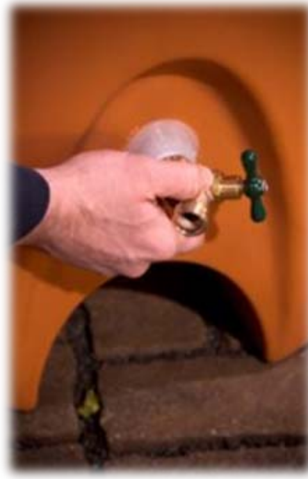
Thread spigot into bulkhead
