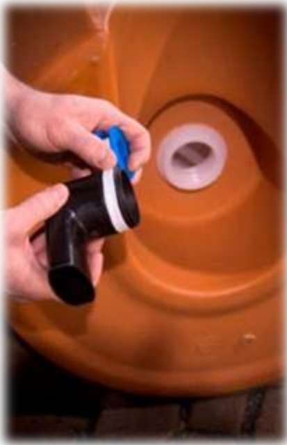
Wrap threads of elbow with Teflon tape
