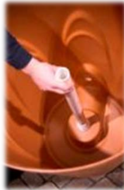
Thread pipe into bulkhead
