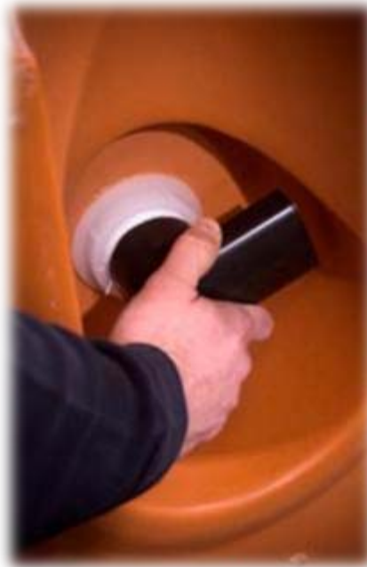
Thread elbow into bulkhead
