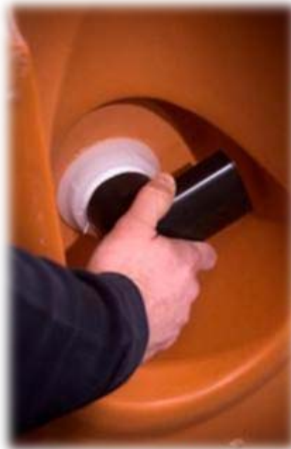
Thread elbow into bulkhead
