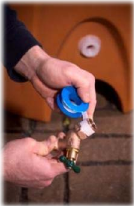
Wrap threads of spigot with Teflon tape
