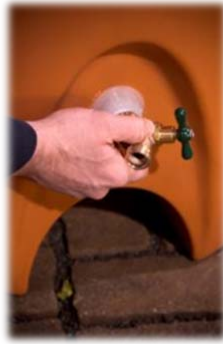
Thread spigot into bulkhead
