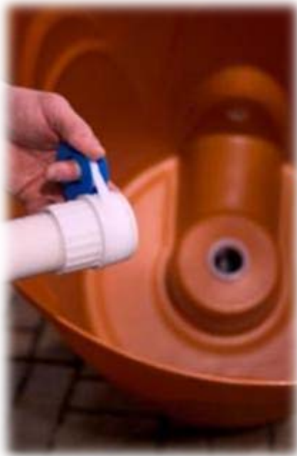
Wrap threads of overflow pipe with Teflon tape
